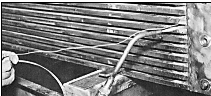
FIG. 28 Brazing repair
